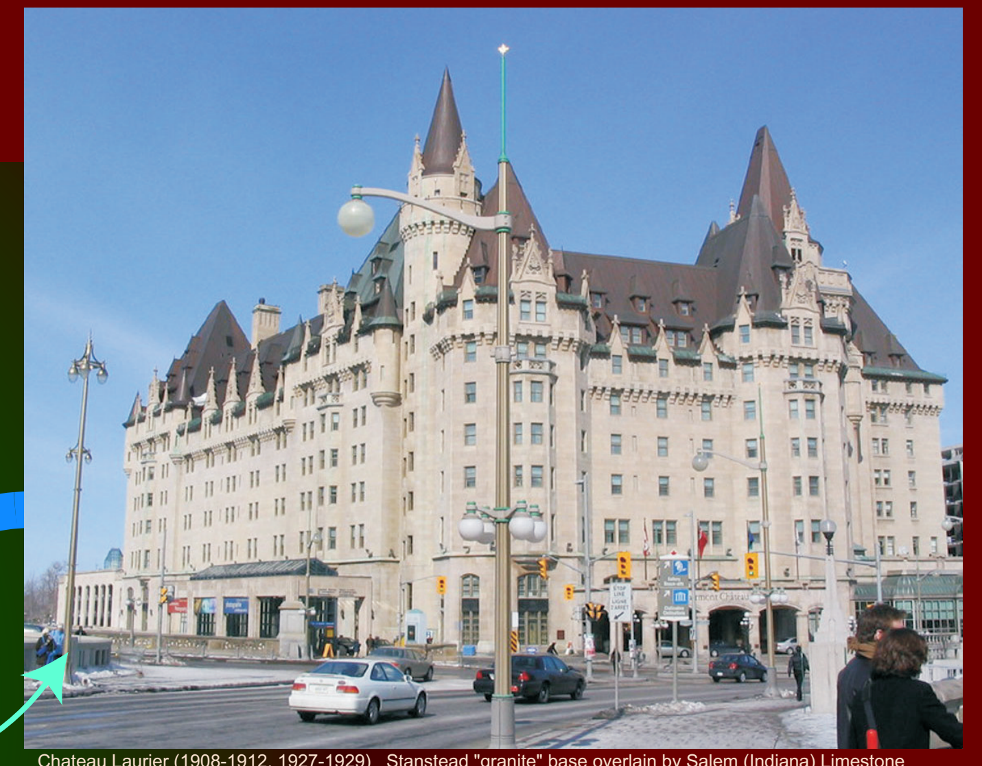
Chateau Laurier (1908-1912, 1927-1929) Stanstead "granite" base overlain by Salem (Indiana) Limestone walls. Copper roof.
